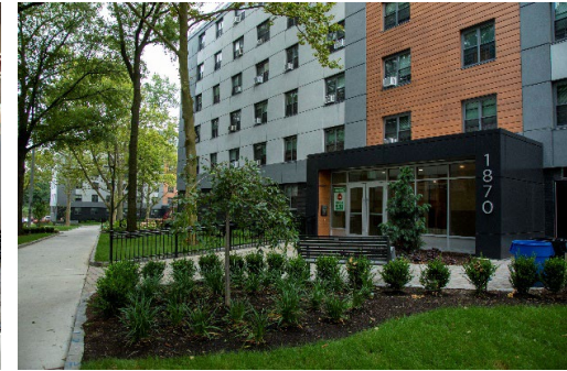
Site improvements at Baychester
