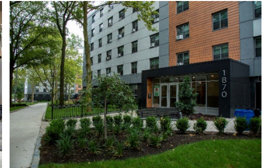
Site improvements at Baychester
