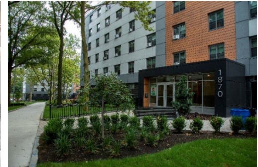
Site improvements at Baychester
