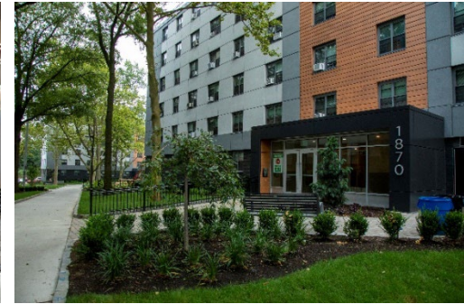
Site improvements at Baychester
