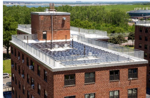
Repaired roof and solar panel system at Ocean Bay (Bayside)
