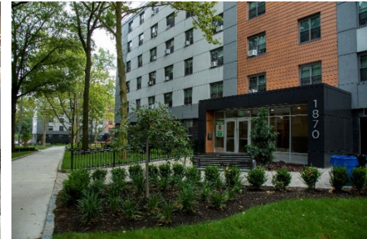
Site improvements at Baychester
